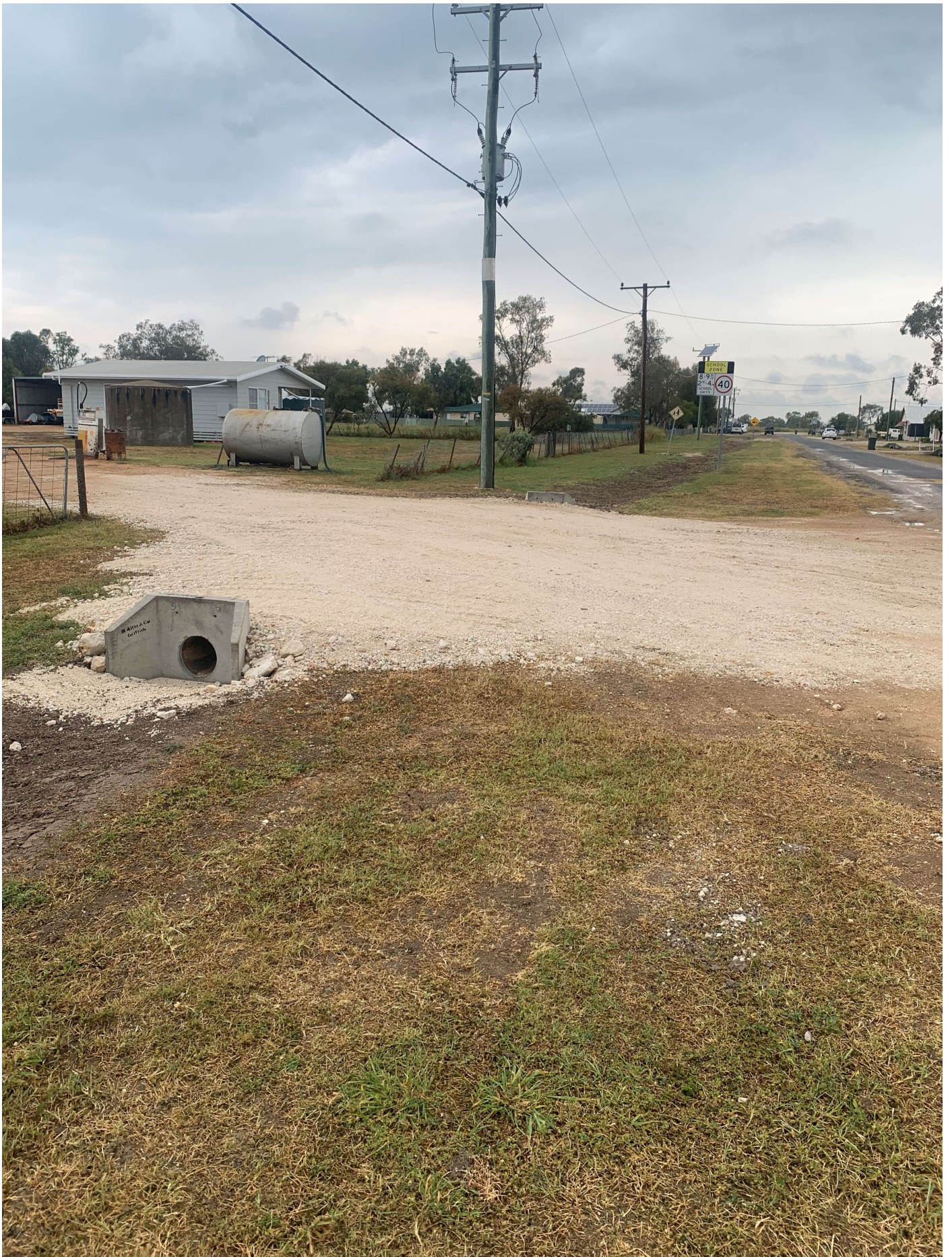
Figure 6 - One of teh new driveway culverts installed.
