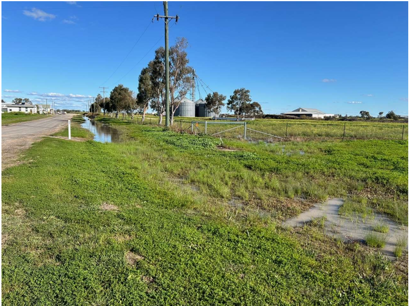
Figure 1 - Before photo of one of the table drains
