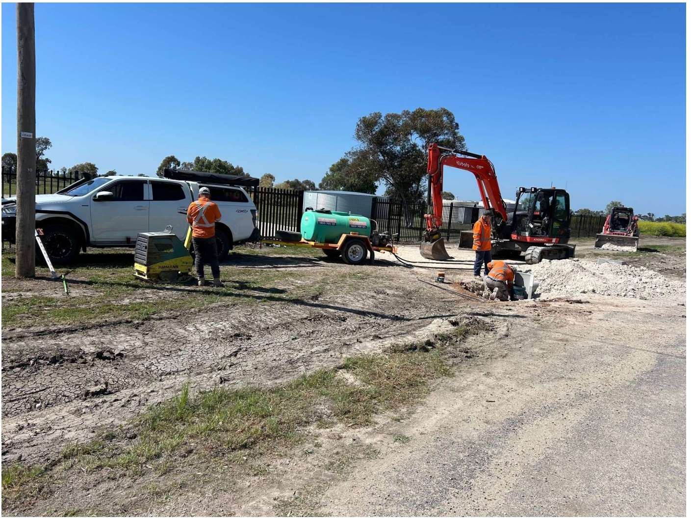
Figure 4 - Works in progress
