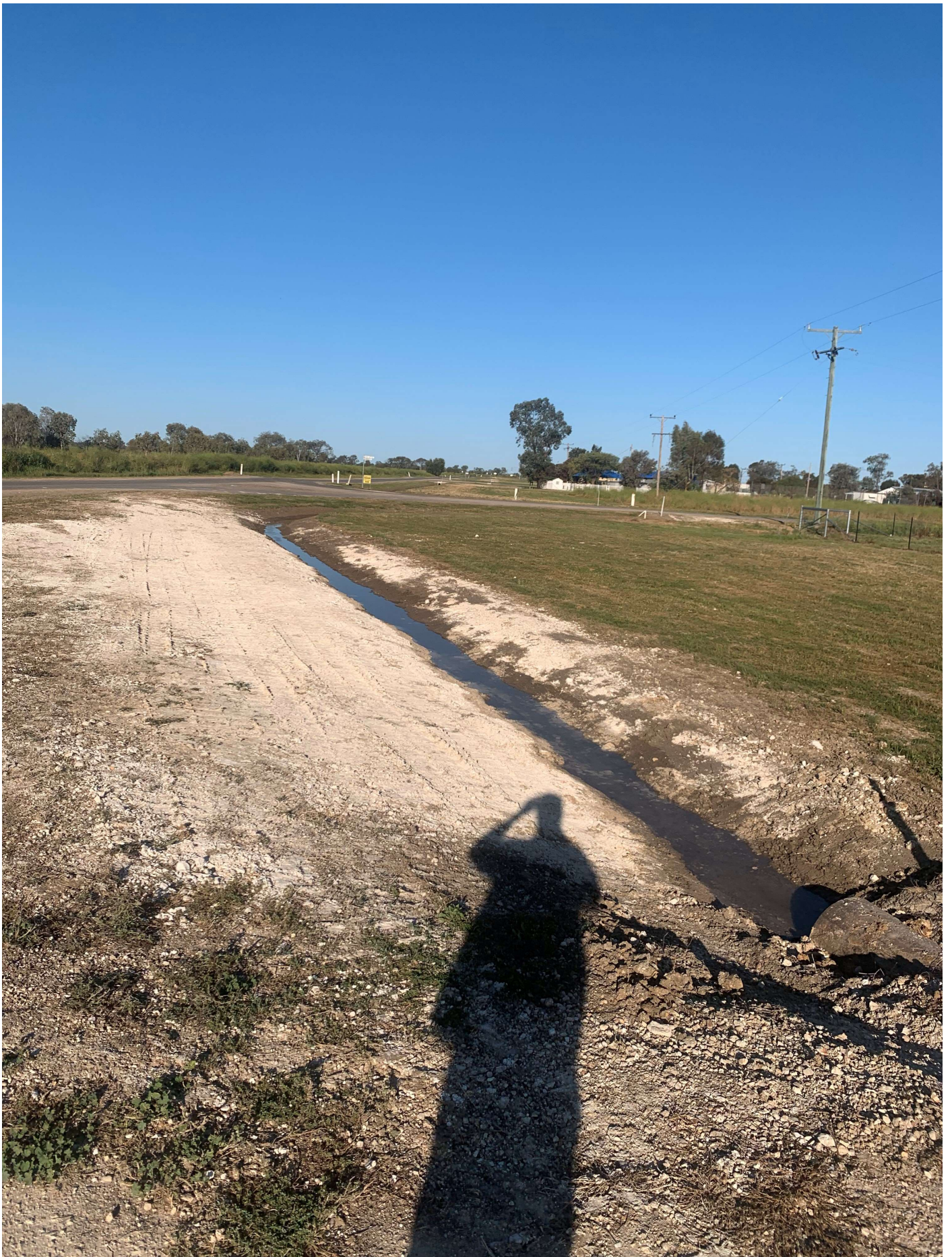
Figure 5 - regraded/ re-excavated drains
