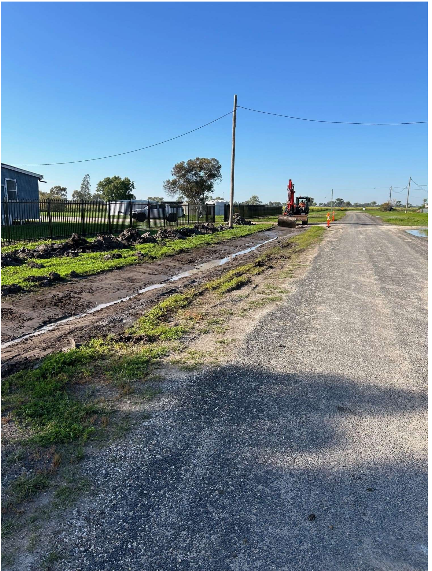
Figure 3 - Works in progress
