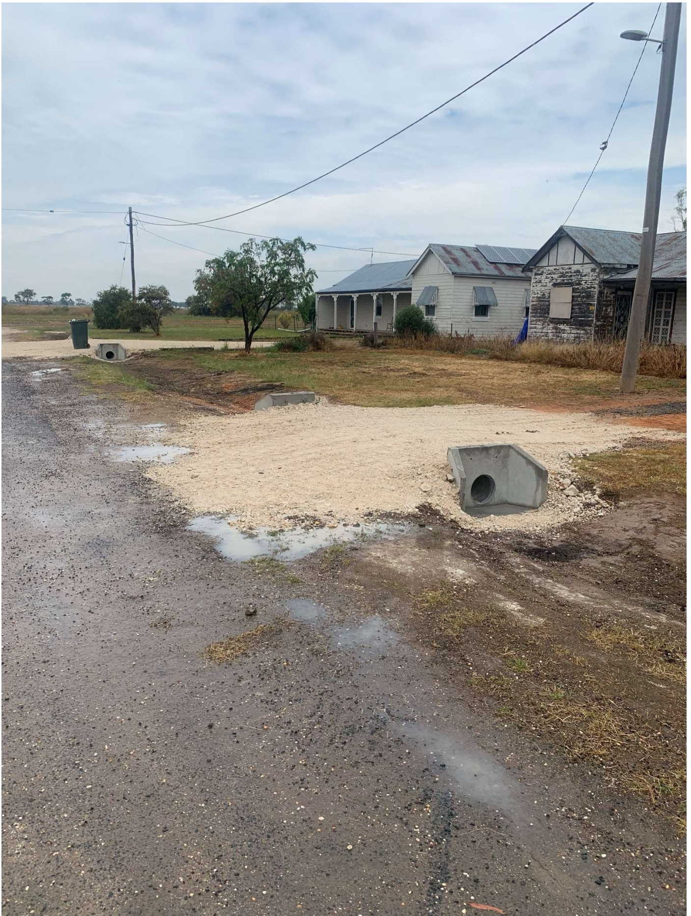
Figure 7 - More of the driveway culverts installed.
